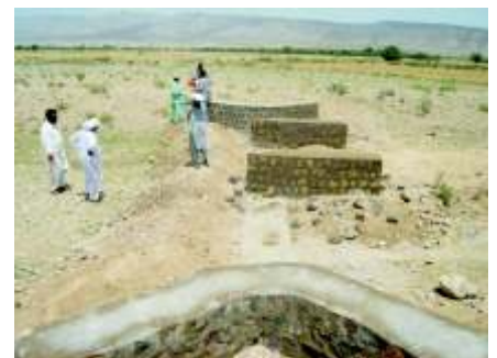
Spate water distribution structures
