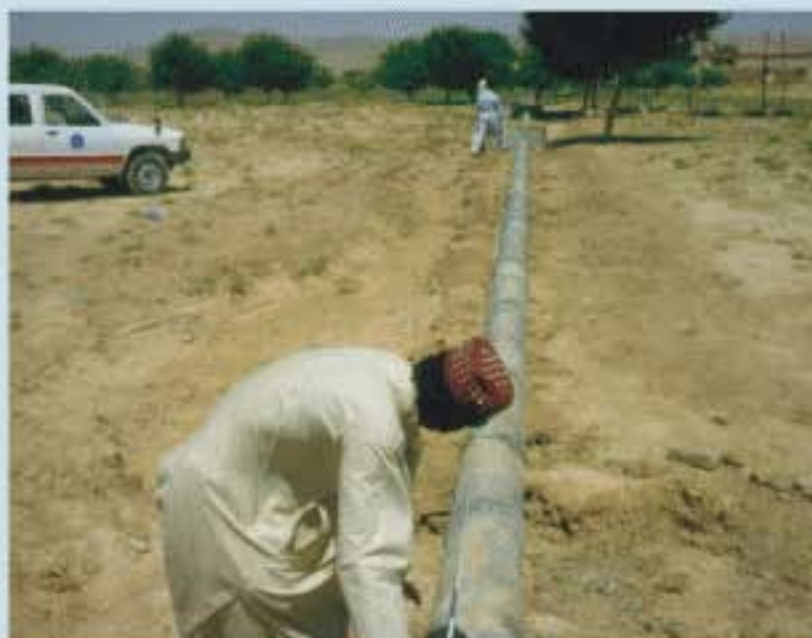
RCC pipe intervention to improve crop conveyance losses
