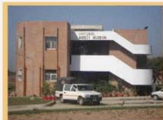
Newly constructed building of "National Insect Museum" at NARC
